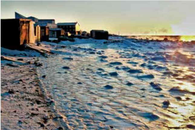
Figure 13. Freeze-up along the waterfront at Iqaluit, November 2011, showing high-tide flooding to the doorsteps of subsistence infrastructure, freezing to form incipient icefoot; even slight changes in sea level, storm climate or ice dynamics could put these buildings at risk, but urban development behind them limits options for setback. Source: Hatcher and Forbes 2015. © 2015 Arctic Institute of North America of the University of Calgary. © Her Majesty the Queen in Right of Canada.
