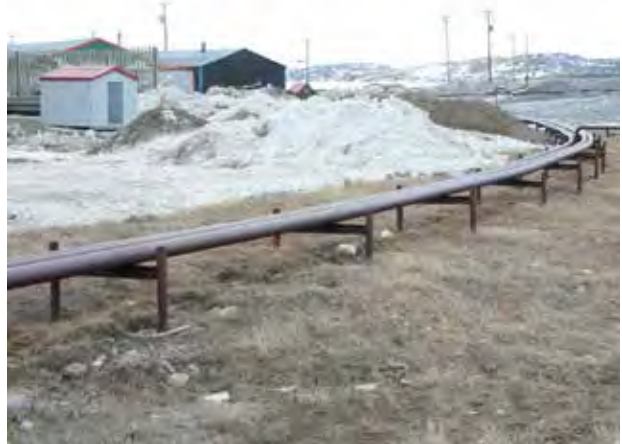
FIGURE 15. Example of oil and fuel distribution pipelines in Iqaluit, NU. These type of pipelines are common in northern communities.
