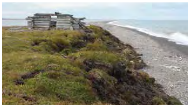
FIGURE 20. Heritage site (1930s cabin) at Nuneluk Spit, Ivvavik National Park, Yukon, 2012. In 1996, the distance from the seaward wall to the top of the cliff was 18.4 m (Forbes 1997); in 2012 it was 0.0 m.
