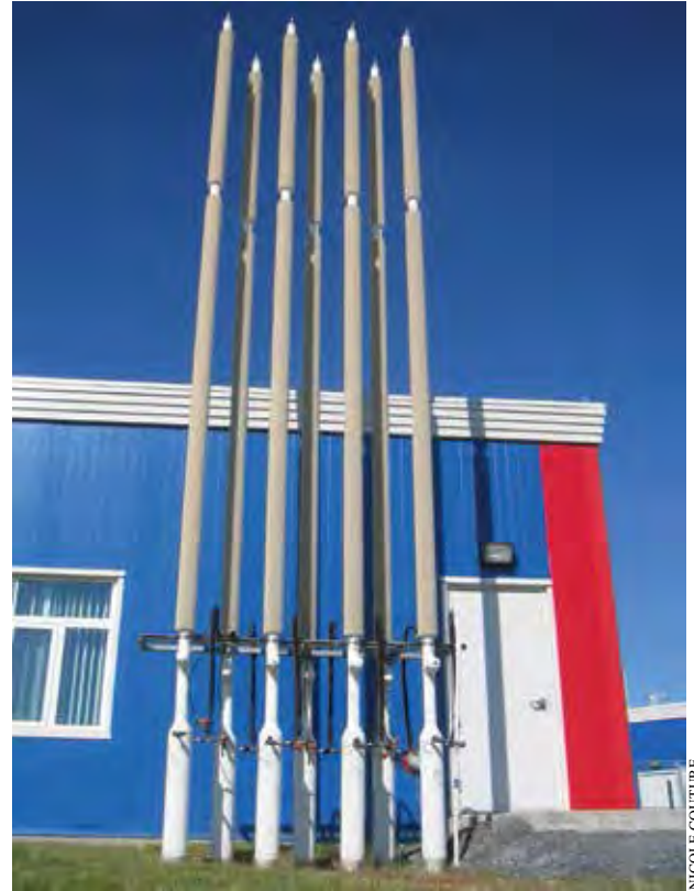
FIGURE 13. Example of thermosyphons installed at the Inuvik hospital. This relatively expensive technique minimizes the impact of the building on the underlying permafrost.
