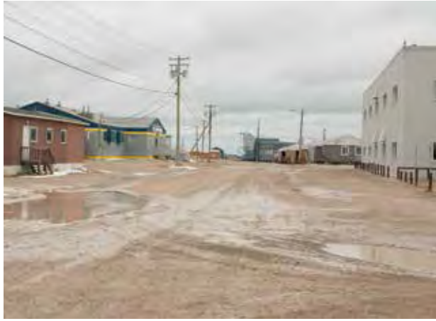
FIGURE 10. Typical road drainage conditions in the ISR and the Kitikmeot region. This example is from Cambridge Bay, NU.
