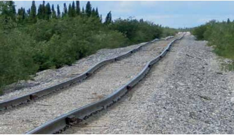
**FIGURE 6.** Damage to rail lines connecting Thompson, MB to Churchill, MB as a result of thermokarst creating subsurface instability
